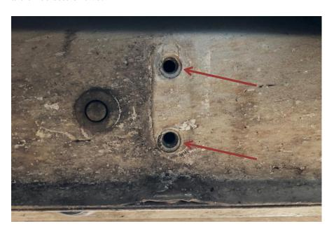
2. Using M8 bolts from hardware kit #27, Thread bolts in and out of inserts to verify threads are clean of debris.
